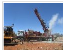
Drilling at Black Cat
